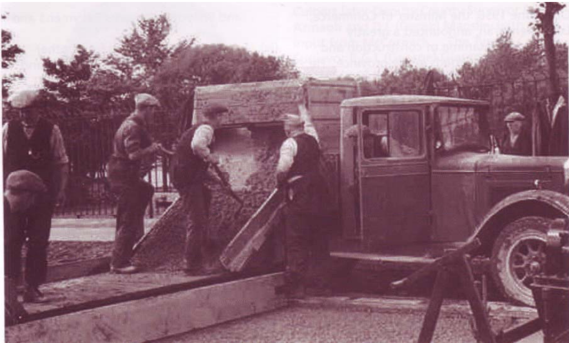
Sydenham Bypass - concrete delivery truck
